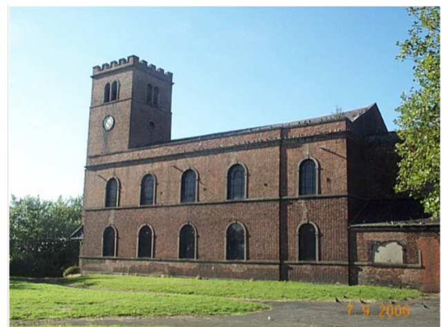
St James Toxteth 2006 showing replaced windows 5
